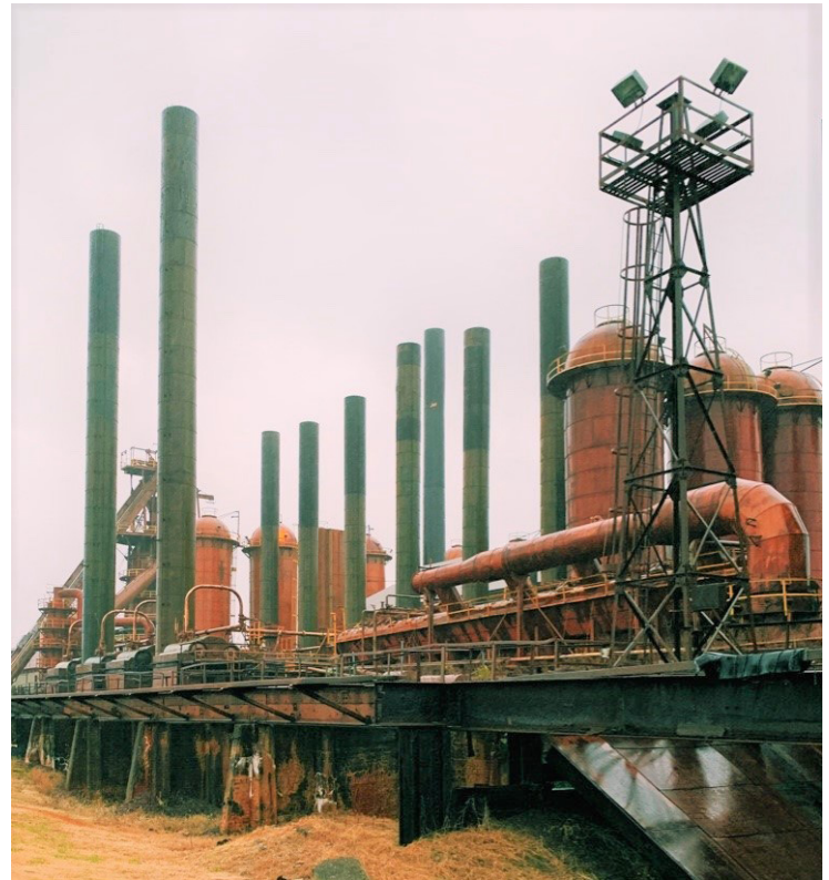
Sloss City Furnaces at Sloss Furnace National Historic Landmark. In the foreground are the stock trestles. Photo taken by Steven Filoromo, 2019.
