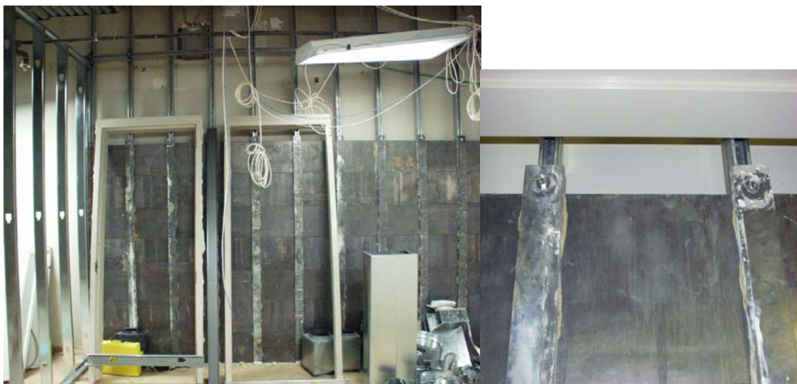
Figure 10. Two Views of the Lead Shielding in the Outer Corridor Wall.
