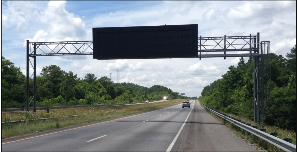
Figure 1-1: Variable Message Sign (VMS)
