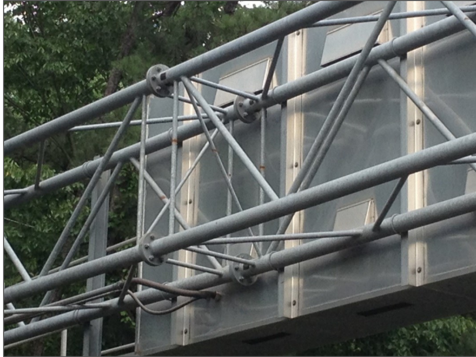
Figure 4-10: Truss Splice Connection of Structure B
