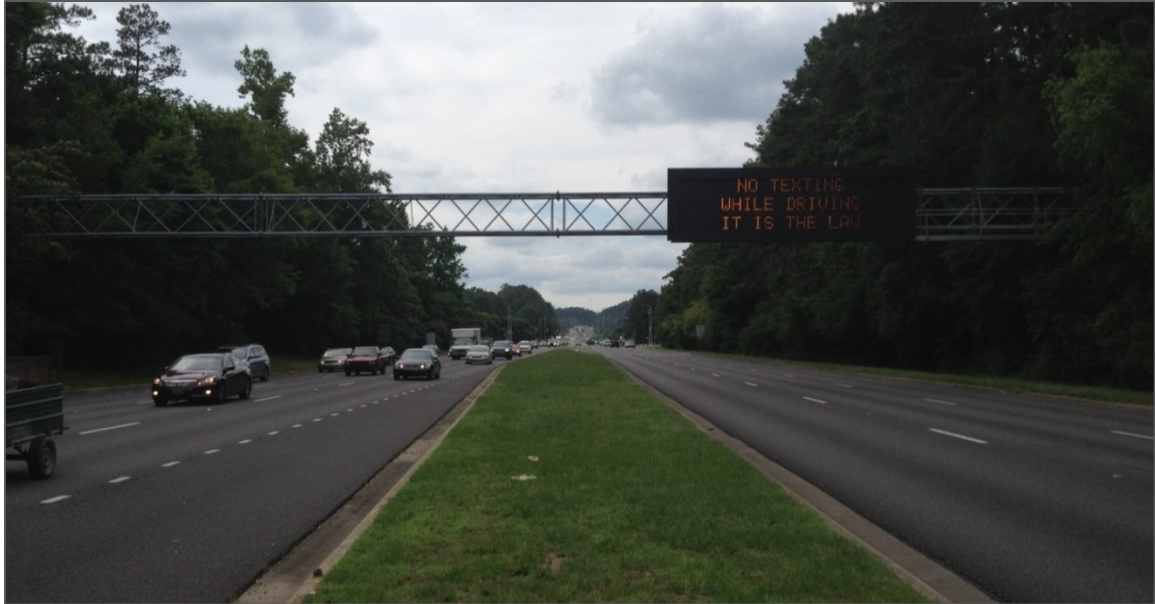
Figure 4-2: Front View of Structure B (Birmingham VMS Structure)
