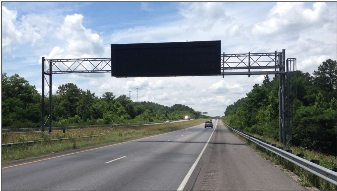
Figure 4-1: Front View of Structure A (Alabaster VMS Structure)
