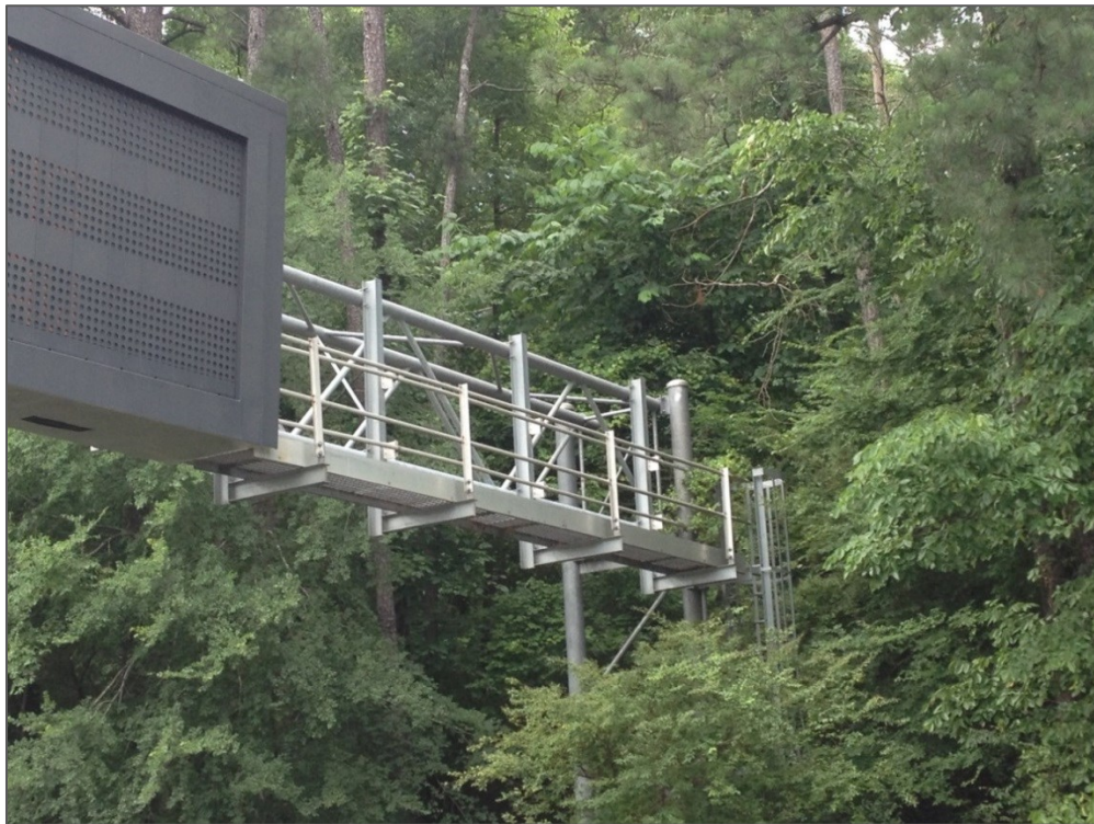
Figure 4-13: Access Ladder and Track of Structure B
