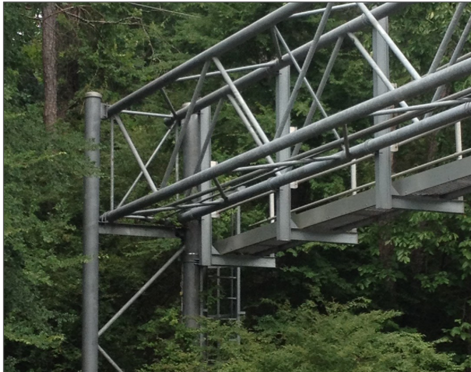
Figure 4-11: Truss to Upright Connection of Structure B
