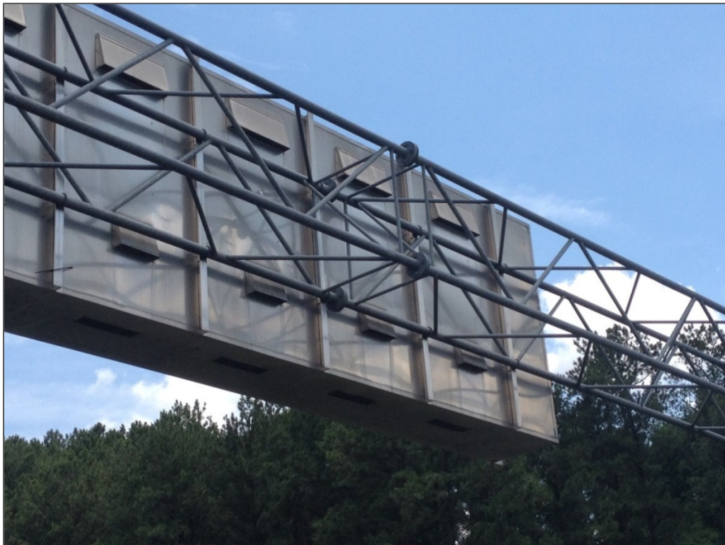
Figure 4-3: Truss Splice Connection of Structure A
