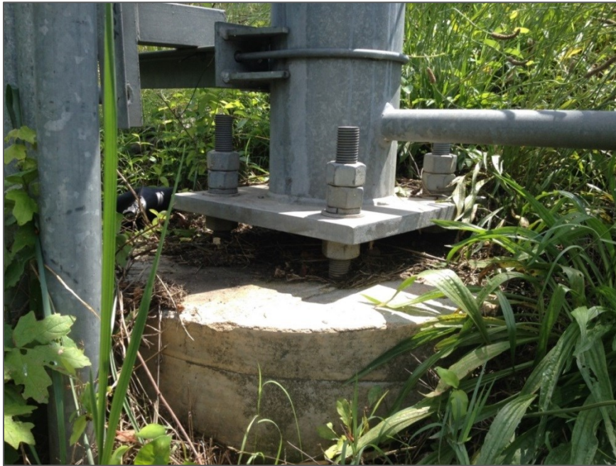
Figure 4-6: Base Plate and Foundation of Structure A
