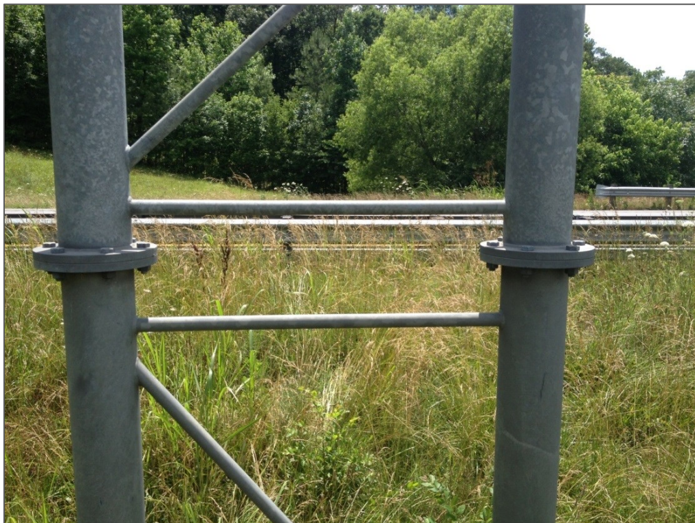
Figure 4-5: Left Upright Splice Connection of Structure A
