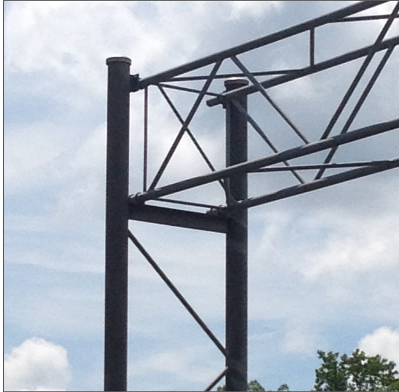
Figure 4-4: Truss to Upright Connection of Structure A
