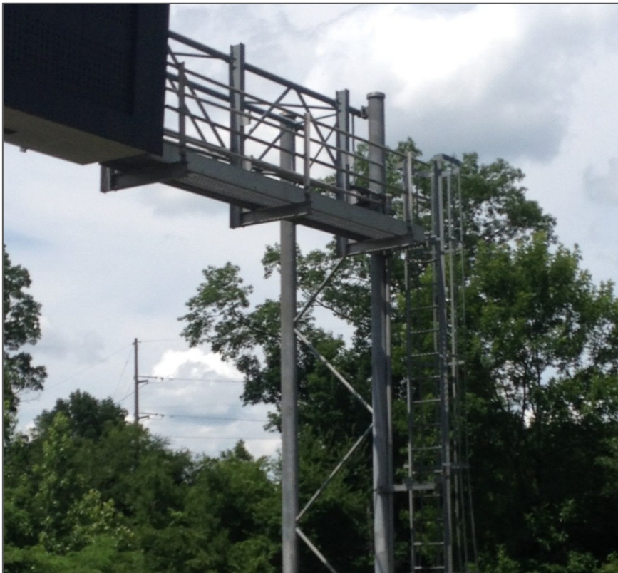
Figure 4-7: Access Ladder and Track of Structure A
