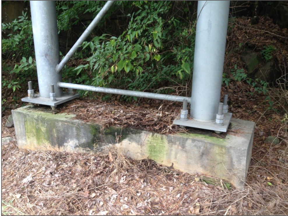
Figure 4-12: Base Plates and Foundation of Structure B
